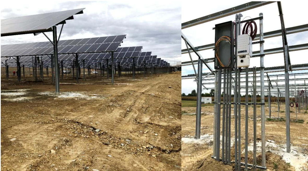
Example solar panel and apparatuses
