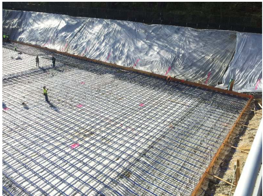
Picture of the West Central Conservancy District's SBR expansion.
