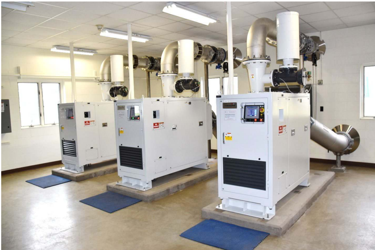
Picture of the City of Plymouth's new Turbo Blowers.
