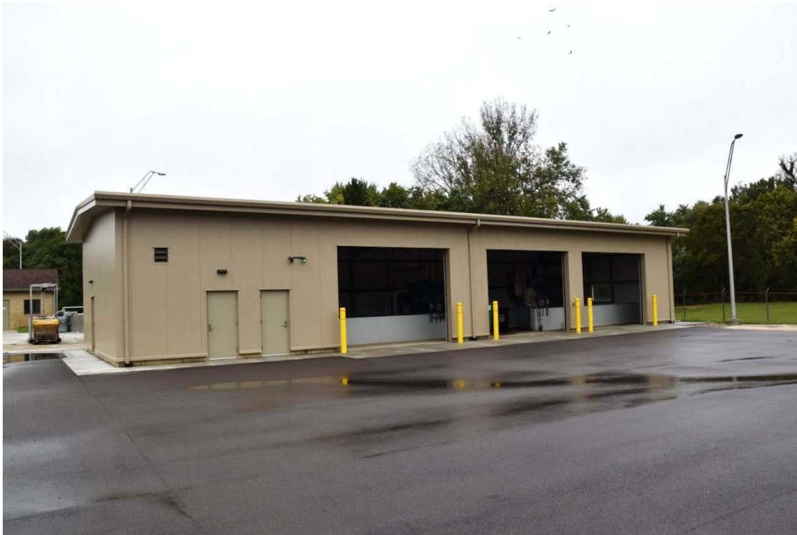
Picture of Plymouth's below ground headworks with a building over the top for freeze protection.
