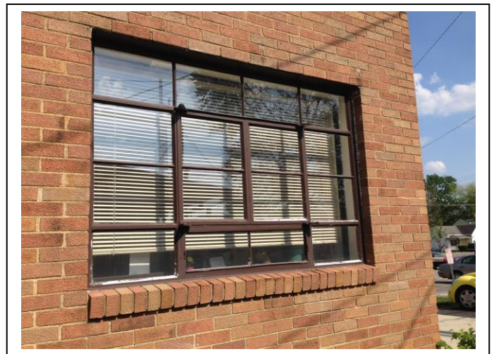
The historic steel windows on the former Napper Hospital were able to be restored as part of the building's 2012 rehab.
