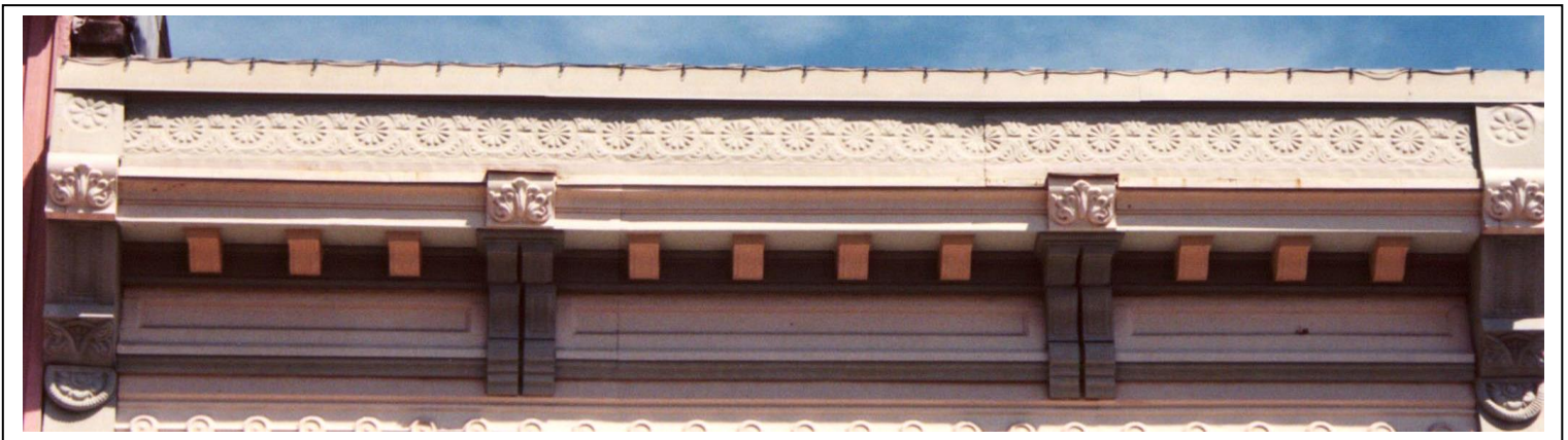
This pressed metal cornice that tops 82 East McClain Avenue was likely made by the George L. Mesker Co. of Evansville, a prominent manufacturer of metal storefronts and other ornament around the turn of the 20 th century.
